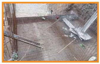
Sikkim: Reinforcement work for Box Culvert Raft in progress at Km. 23+270
