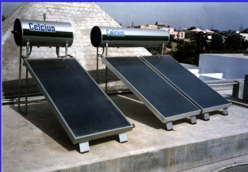
DOMESTIC SOLAR WATER HEATERS
