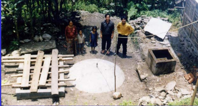
Family size ( 2 Cubic Meters) biogas plants in rural area of Sikkim.
