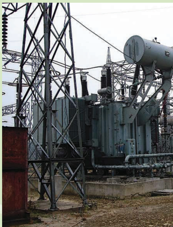
Augmentation of 220/132 KV 2x50 MVA SS in Mariani to 2x100 MVA (Transformer I & II) in Jorhat district of Assam
