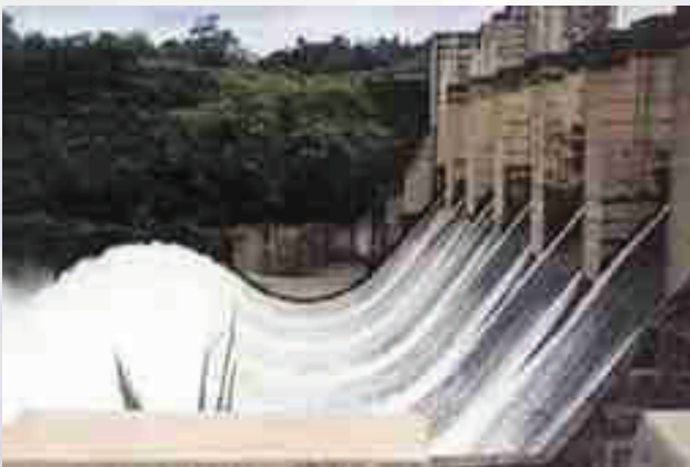
Khandong Dam, Kopili H.E. Project (275 MW), Assam
