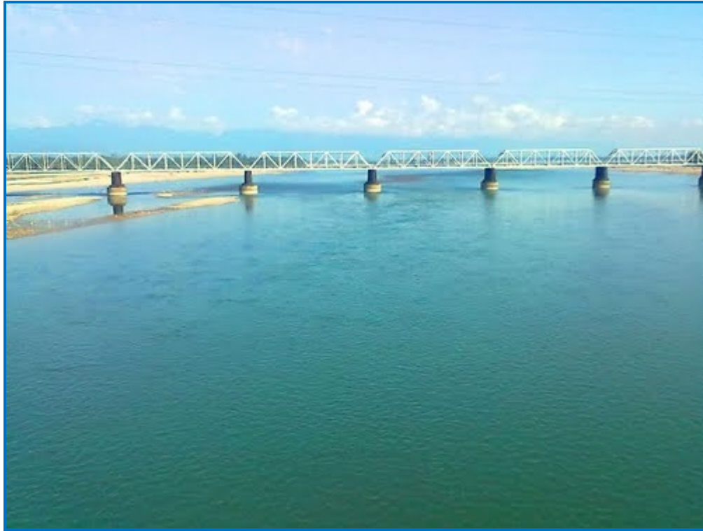
Fig. 5.6: Subansiri River, a view from NH52 at Balijangoan
